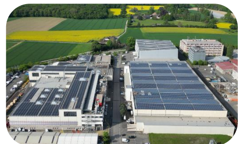
Figure 5. Aerial view of Hitachi Energy’s rooftop PVs
