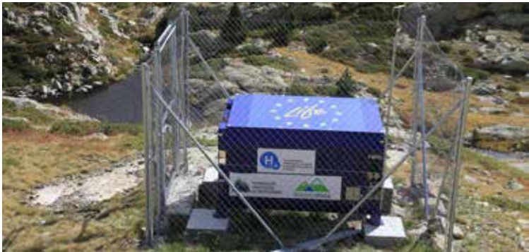
Hydrogen Storage at Bachimaña´s hut.
