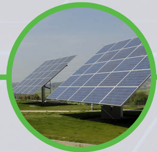
DEGER 1. 5,5 kWp Panel policristalino Polycrystalline cells DEGER 2. 5,25 kWp Panel monocristalino Monocrystalline cells
