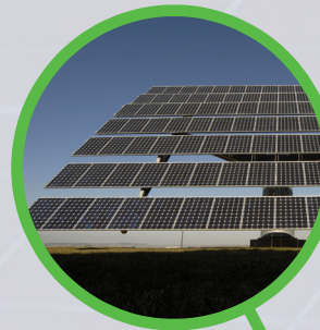
ADES. 23,5 kWp Panel monocristalino Electrical substation
